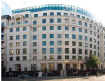
ONE LOTHBURY DEVELOPMENT IN CITY OF LONDON
